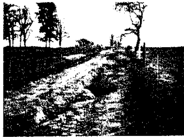
Frequent lane use and poor layout design lead to excessive erosion problems.
